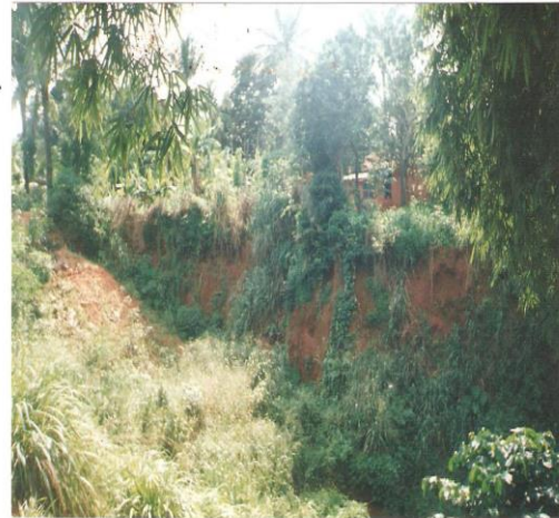
Plate 2: A House Threatened by Gully Erosion in Chikun LGA Source: Field Work, 2016
